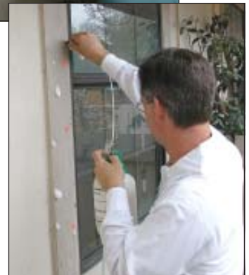
Top two photos: Using the AED-2000 to listen for termite activity. Bottom photo: Treating the drywood termite gallery with a foam termiticide. (Photos: Doc Nichols).
